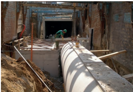
Construction of a pipe gallery and utility network displacement at la Pitié-Salpêtrière Hospital in Paris (75)
