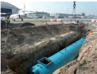
Installation of hydrocarbon separators in restricted area in Le Bourget Airport (93) IGREC INGENIERIE project manager and representative
